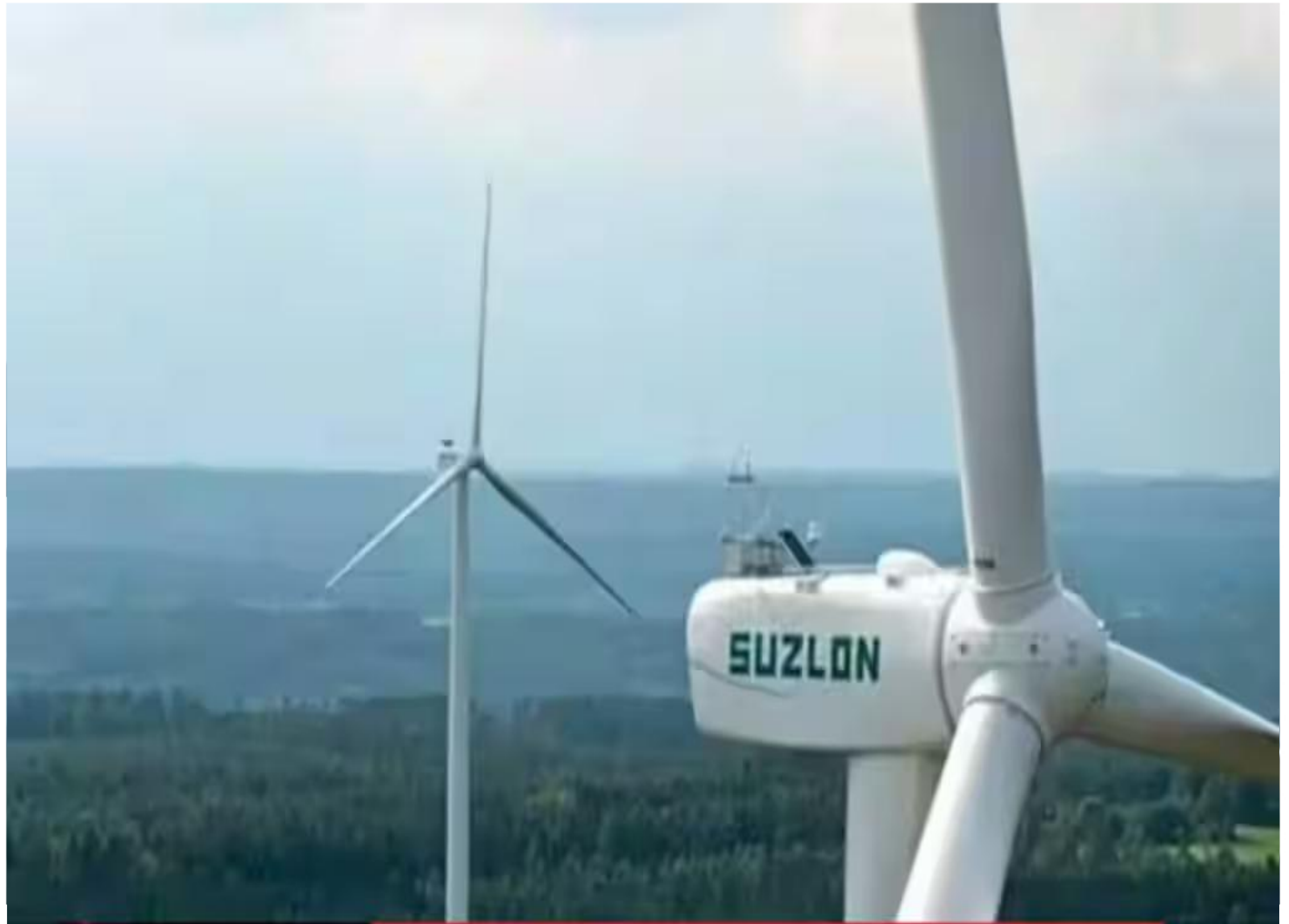
Suzlon Group announced a new order win for the development of a 193.2 MW wind power project for The KP Group.
